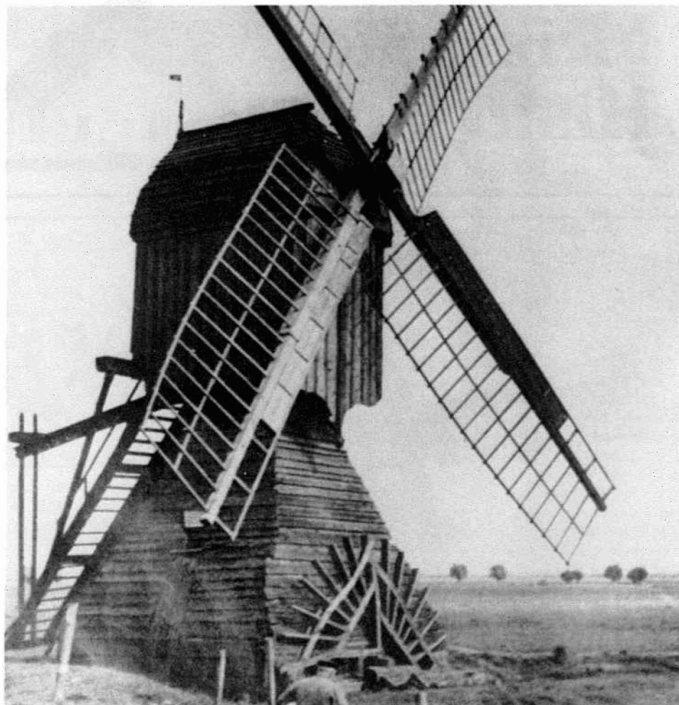
This mill is of hollow post mill (Wipmolen) design and was located at one of the Mennonite settlements in Prussia. The sails were faced into the wind by means of the tail pole which can be seen extending from the rear of the cap. This mill was likely used for pumping water, that is, for drainage, and not for grain milling. (Photo courtesy Mennonite Heritage Centre)
