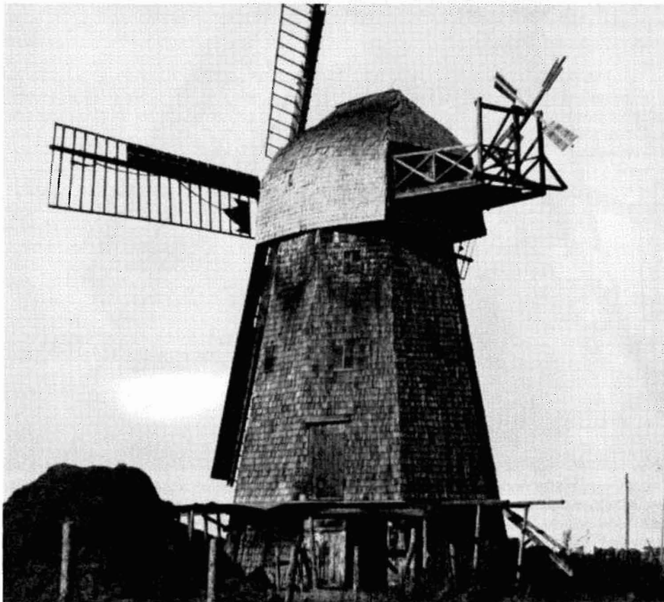
A side view of the Rosenort (Scratching River) Windmill. It was of standard smock mill design. The windmill cap rotated on a metal track. Any change in wind direction would cause the "fan" to turn, which would then move the whole cap until the sails faced directly into the wind. (Photo courtesy Provincial Archives of Manitoba)
