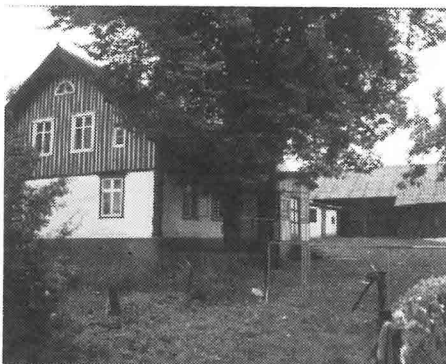
One of the building styles used by Mennonites in the Zeyersvorderkampen area. The house and barn are built in the shape of a T. Because the farmland is about six feet below sea level, flooding was a constant danger as can be seen in the photo. The buildings were built on a mound of soil to protect them in case of a flood. Photo credit: John Friesen, CMBC.
