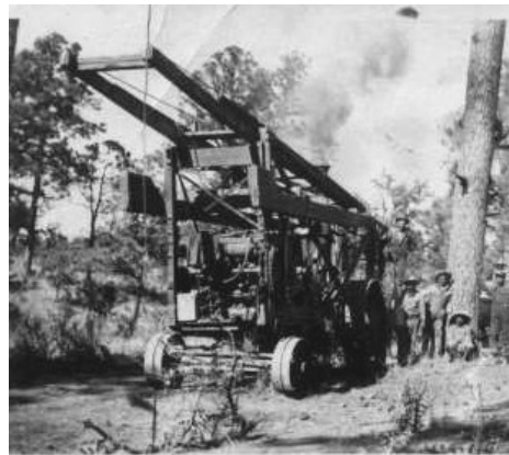
Steam powered well drilling machine traveling along a road through a treed area. Six men stand beside the machine posing for a photo. A wagon with a water tank is behind them. Photo: MHC Collection 592:27
