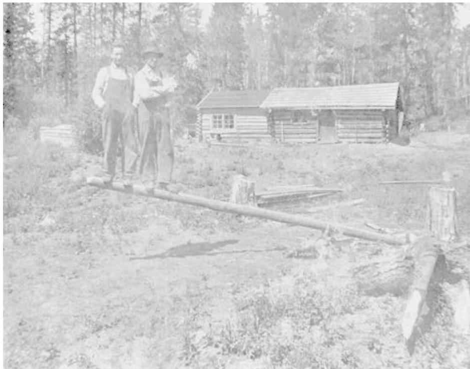
Clearing land in the Nechako Valley near the Vanderhoof settlement. Brothers Abe Suderman and Jake Suderman stand on a long-pole lever and use their combined weight to loosen a stump. Photo: Courtesy of Harold Suderman.
