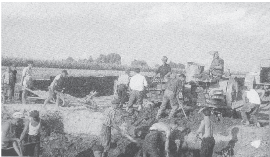
Yugoslav workers making adobe bricks for reconstruction after the flood.
