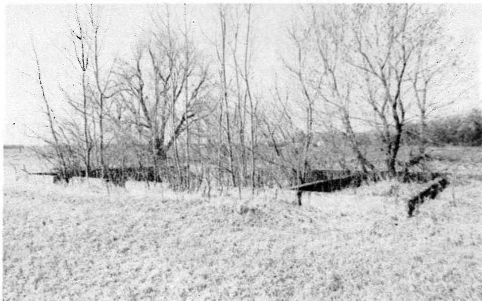
The existing basement remains of the meeting house for the Herold Mennonite congregation, Morden, Manitoba. Photo courtesy of Karl Klaassen, Kelowna, B.C.
